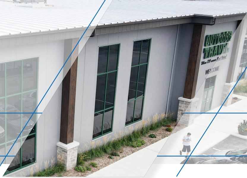
The Metl-Span CF Santa Fe panel has a flat exterior profile with a heavy, embossed stucco texture that mimics the look of a masonry stucco finish but with the added value of an insulated metal panel. The profile is flush with the warmth of an old-world finish, providing a visually pleasing building.
