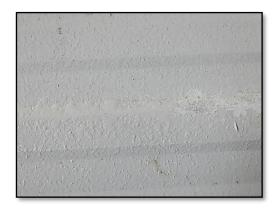
are a white chalky powder or raised texture in the paint. As the stain becomes more acute, the paint will delaminate from the panel surface and the final stage will be red rust.
